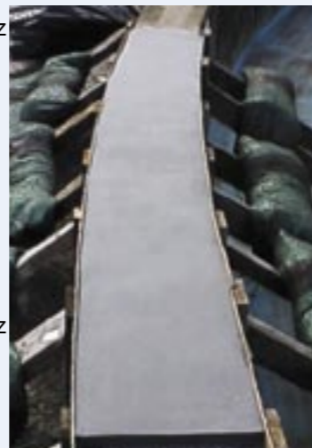
Rebuilding and re-reinforcing with Fixmaster® High Performance Quartz
