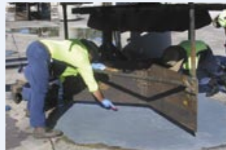
Applying Fixmaster® High Performance Quartz
