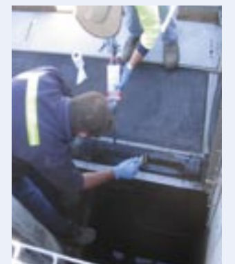
Applying Fixmaster® Rapid Rubber Repair
